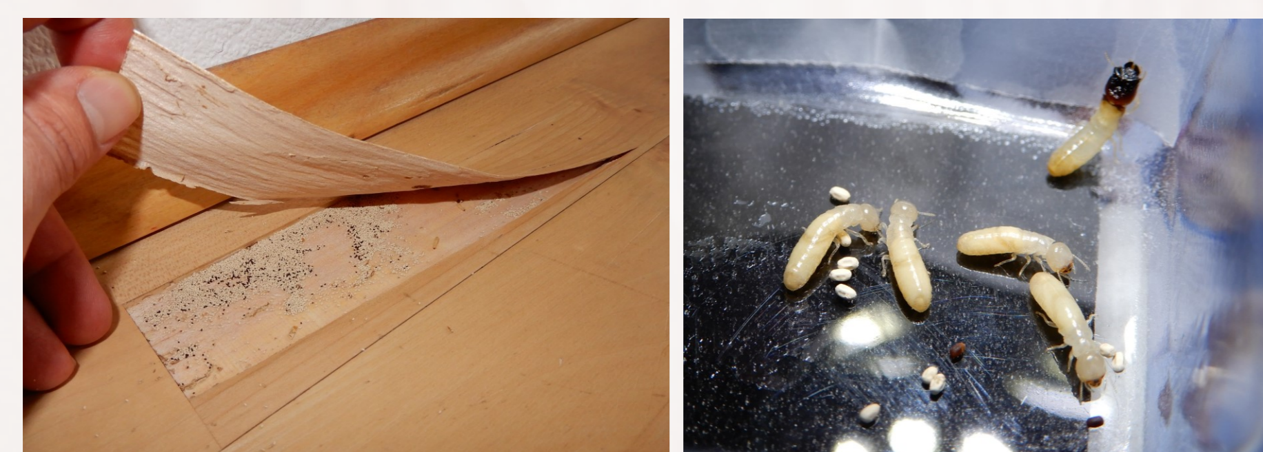
Figure: 4-5 Drywood termites at a wood laminate floor (2018 München)
